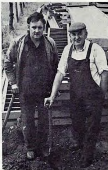
AND ON THE GROUND... with the last joint finished John Parry ( jointer ), left, and Cyril Griffiths ( jointer's mate ) relax for a while.
